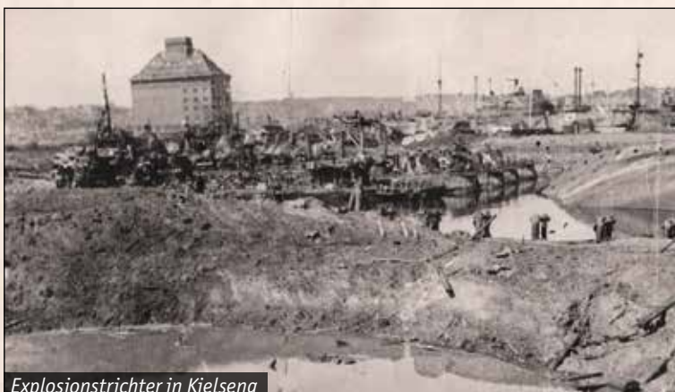
Explosionstrichter in Kielseng
